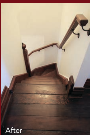
Above: Addressing hazardous stair elements such as missing treads and handrails is a typical requirement under the By-Law. See Section Three for more on stairs.
