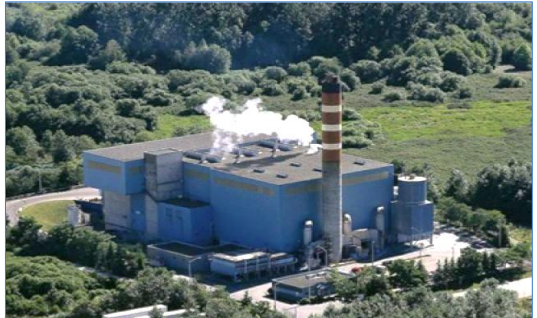
Metro Vancouver Waste to Energy Facility (Burnaby)
