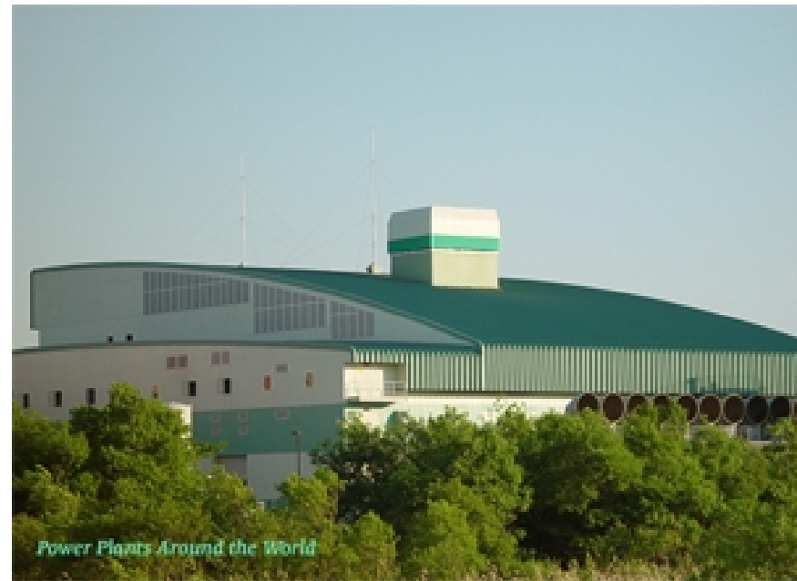
Mutsu Gasification facility in Japan
