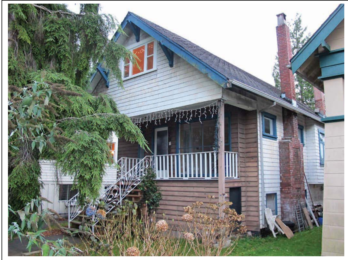
Front and West Side of Birnie House, 3182 West 3 rd Avenue
