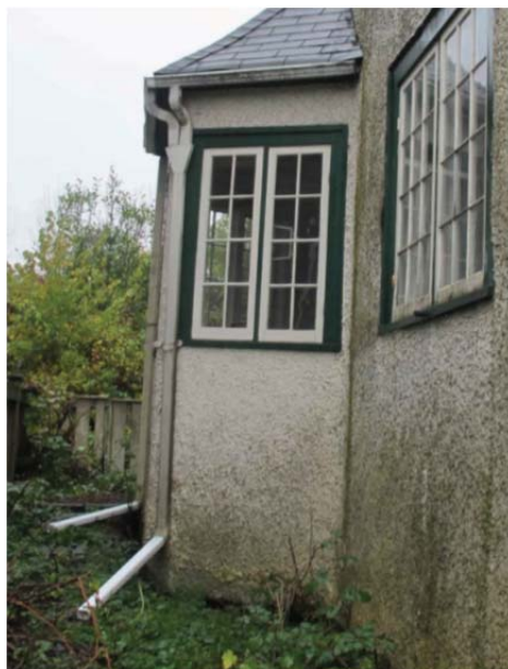
Photo 2: West side bay window
