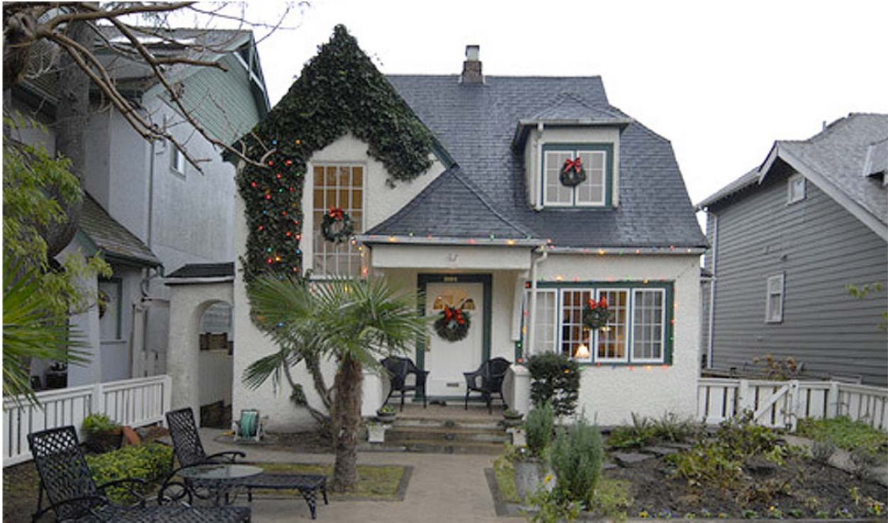
Photo 1: The Muller House at 3091 West 3 rd Avenue, looking north from West 3 rd Avenue
