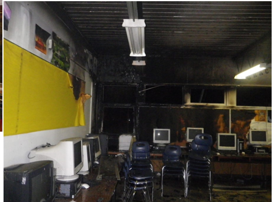
Eric Hamber Annex - 2011 ($410,000 damage)
