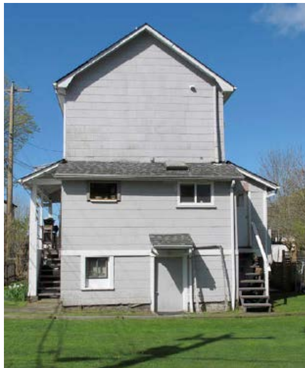
Photo 6: The east side of 3308 Ash Street (looking west)
