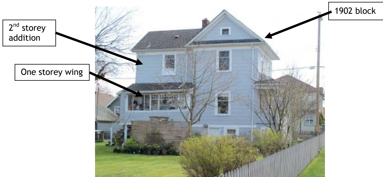
Photo 7: The heritage building is believed to have been built in three phases: (1) a small, original two storey portion (the 1902 block); (2) a tiny one storey wing added shortly thereafter; and (3) a second storey addition added to the wing, possibly in 1945 (see the maps in Appendix B).
