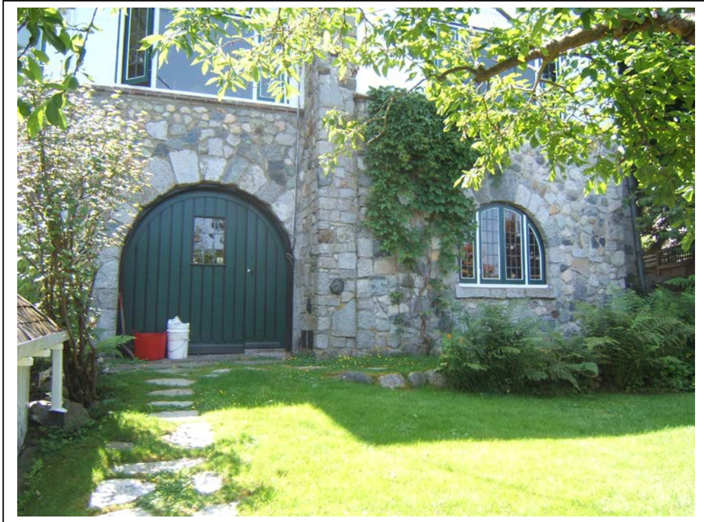
4629 West 2 nd Avenue - Campney House Door and Window Detail at Lower Rear
