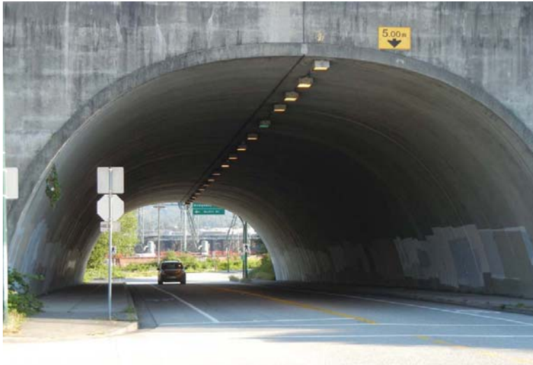
Figure 2: Bridgeway Street Tunnel - existing condition
