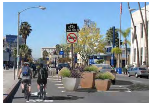
Figure A-12: Separated Bike Lane on 3rd Street in Long Beach, California
