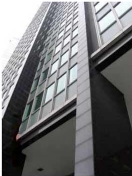
Figure 3: Detail of granite fins
