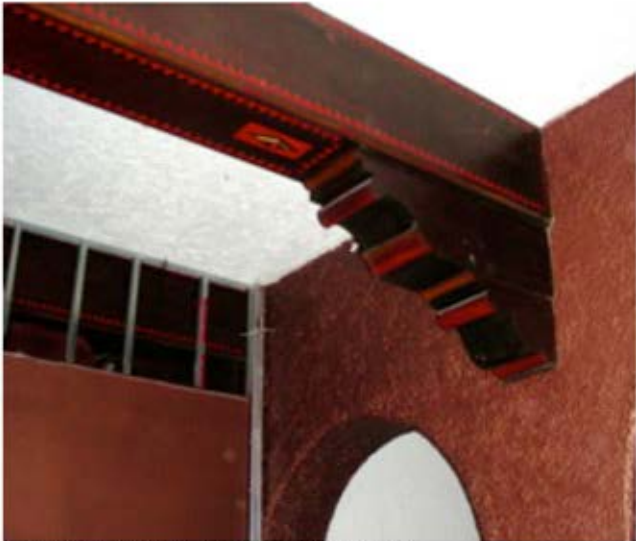
Figure 7: Detail of painted Lobby beam
