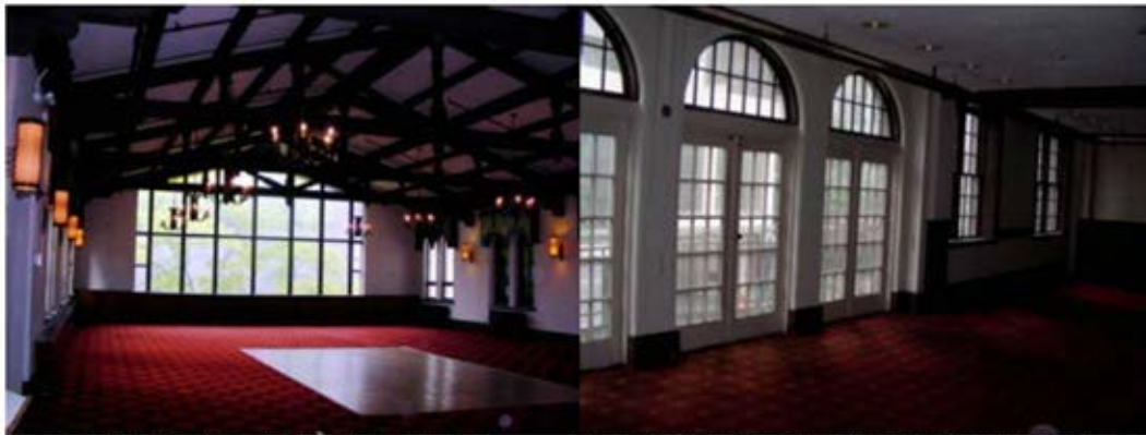
Figure 7: Upper Floor Dining Room trusses
