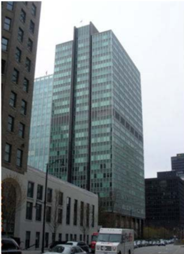
Figure 2: View from Cordova Street
