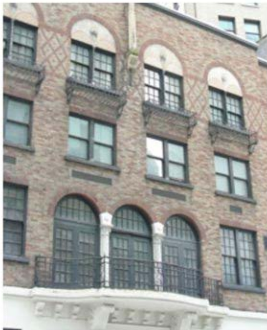
Figure 3: Detail of West Hastings façade
