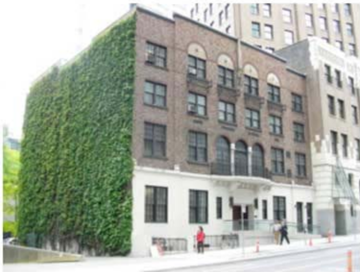
Figure 2: View of West Hastings façade
