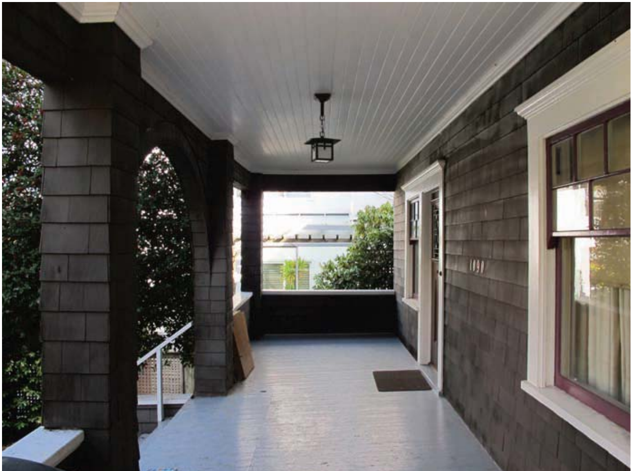
Photo 6: View of the front porch, looking north east. Everything is original except the front stairs. The building at 1480 Comox Street is visible in the background.
