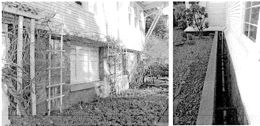
Foundation walls built with granite rubble stone and visible on the south facade (left); open drainage system on the north elevation (right).
