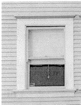
Original double-hung wood sash window on the west elevation.
