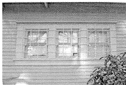
2-over-1 double-hung windows on the north elevation with metal security grills.
