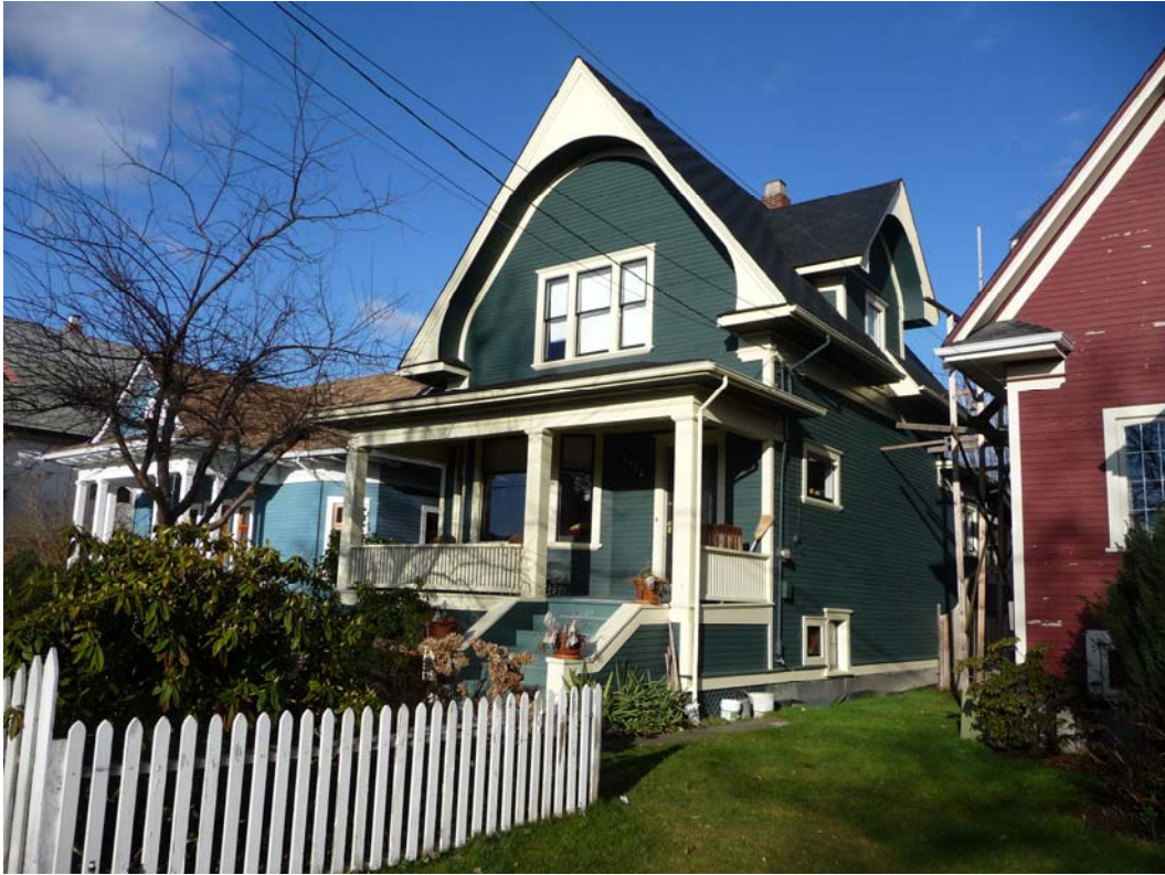
Imrie House, 4446 James Street
