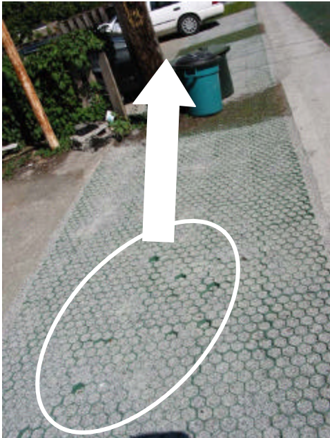
Figure 6.8 Gravel 'hydro-excavation'
