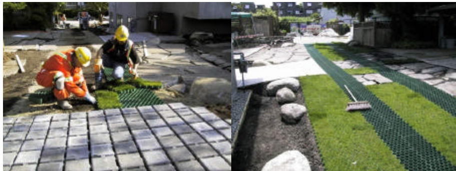
Figure 5.6 Pre-grown grass placement
