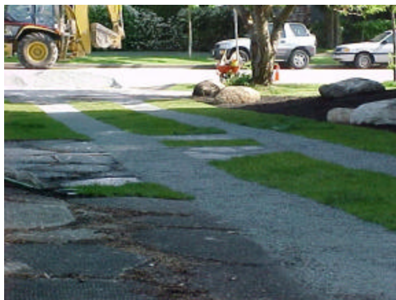
Figure 5.3 Gravel-filled Golpla Driving Strips
