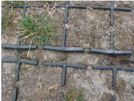
Figure 4.6 Geoblock joint strains
