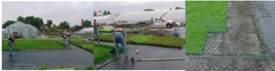
Figure 5.5 Pre-grown grass removal
