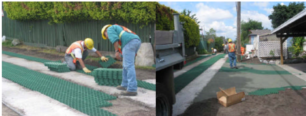
Figure 6.2 Golpla Placement
