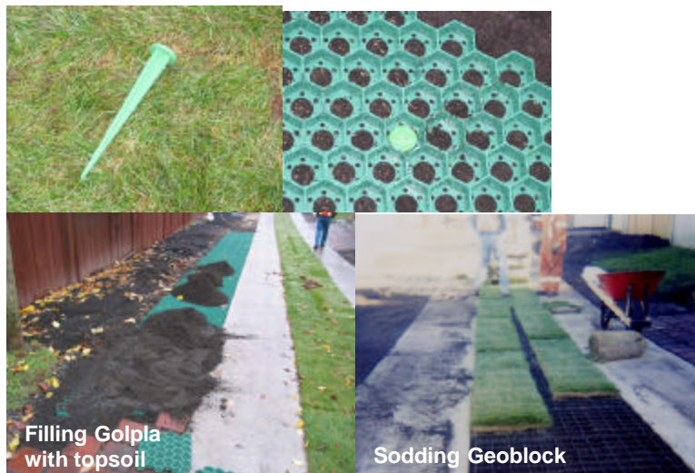
Figure 4.3 Structural Grass Construction
