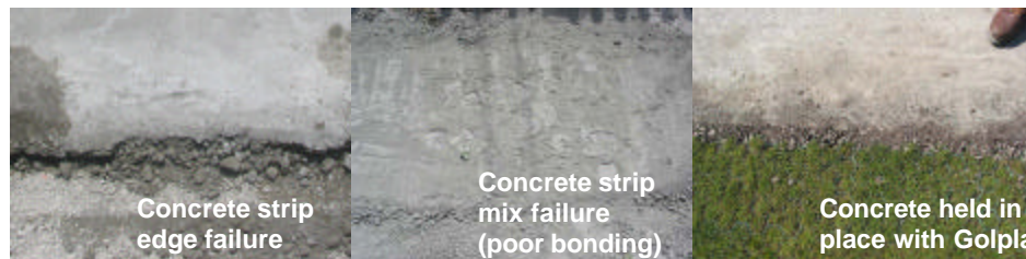
Figure 6.4 Dry mix driving strips
