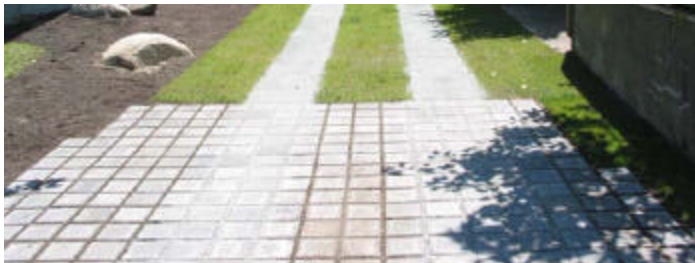
Figure 5.9 Permeable Paver Lane Entrance
