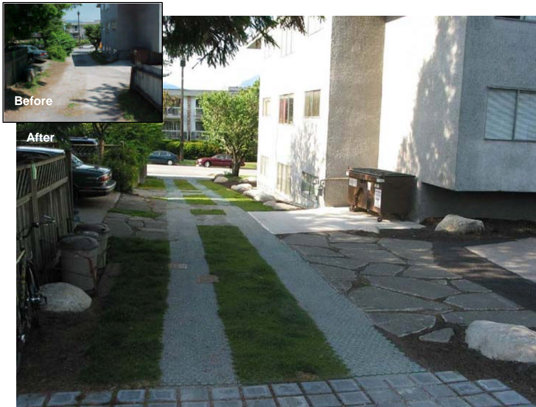
Figure 5.2 Second Country Lane Improvement
